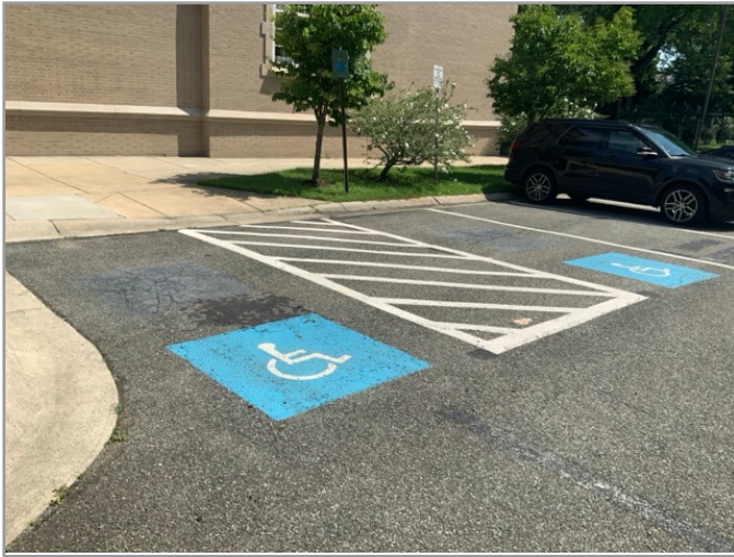
OVERVIEW OF ACCESSIBLE PARKING AREA
